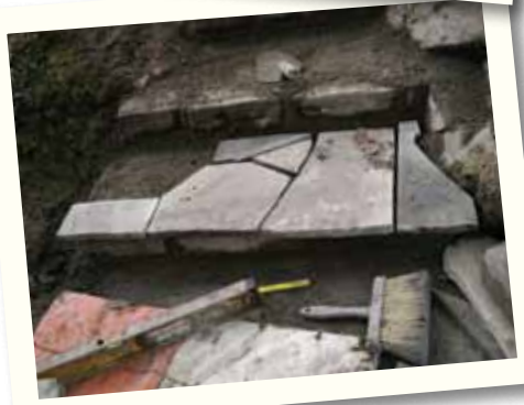
Top: Abkhazi Garden is the recipient of a 'Canada 150 Garden Experience' designation, awarded by the Canadian Garden Council in collaboration with the Canadian Nursery Landscape Association. Photo credit Dennis Robinson. Bottom: Stonework to restore the stairways reusing original stones. Photo credit Andrew MacKinnon.
